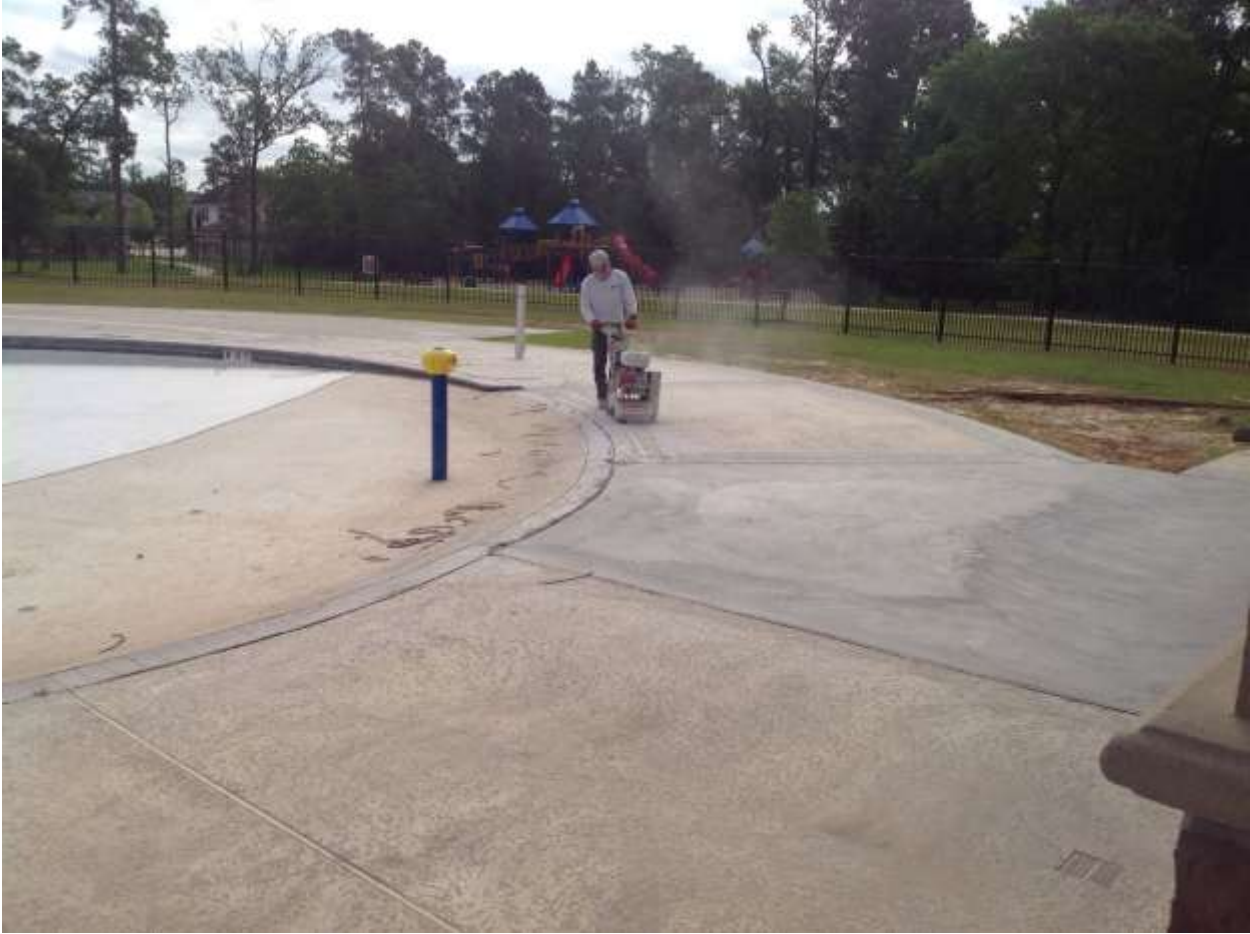
Description: Poured the concrete for various pool deck panels.
